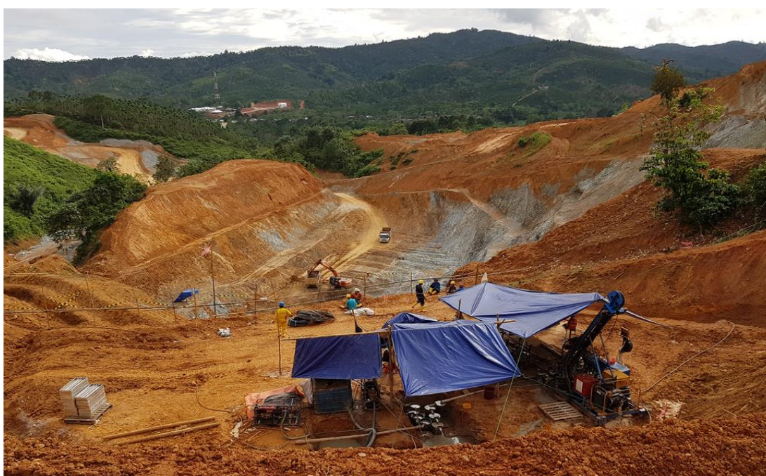
FIGURE 1: Diamond Drilling at Talang Santo
