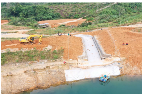
Construction of Talang Santo Pit Spillway
