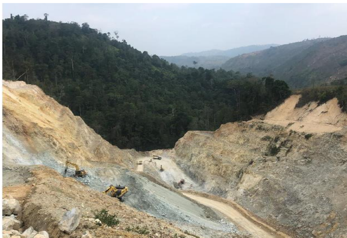
Figure 1: Way Linggo Open Pit looking east
