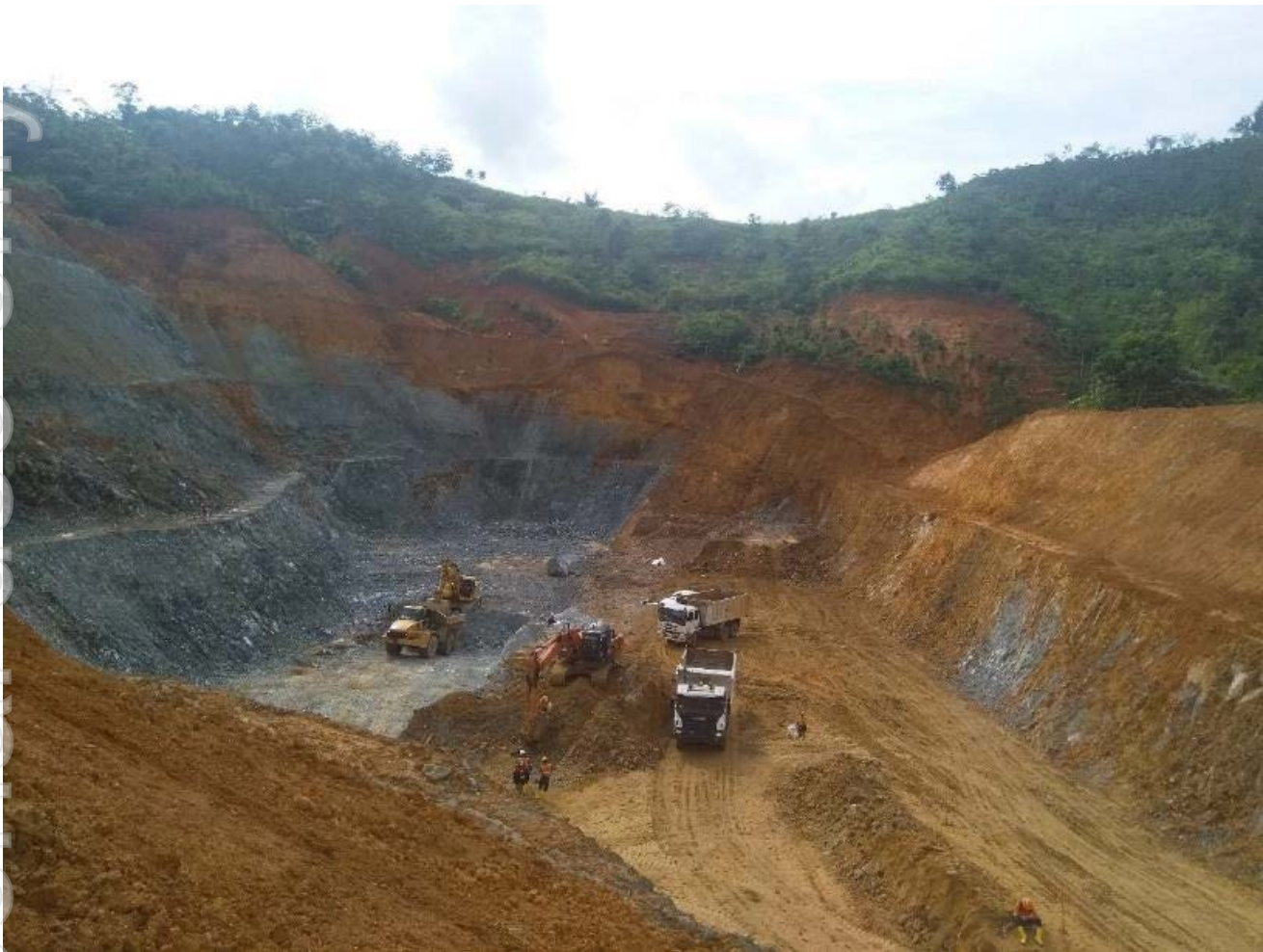
Figure 2: Talang Santo Stage 3 Pit March 2019
