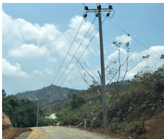
Figure 2: New powerlines erected
