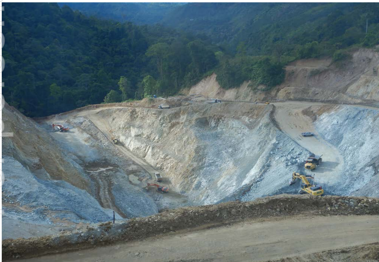
Figure 1: Way Linggo Open Pit at 31 December 2018, looking south
