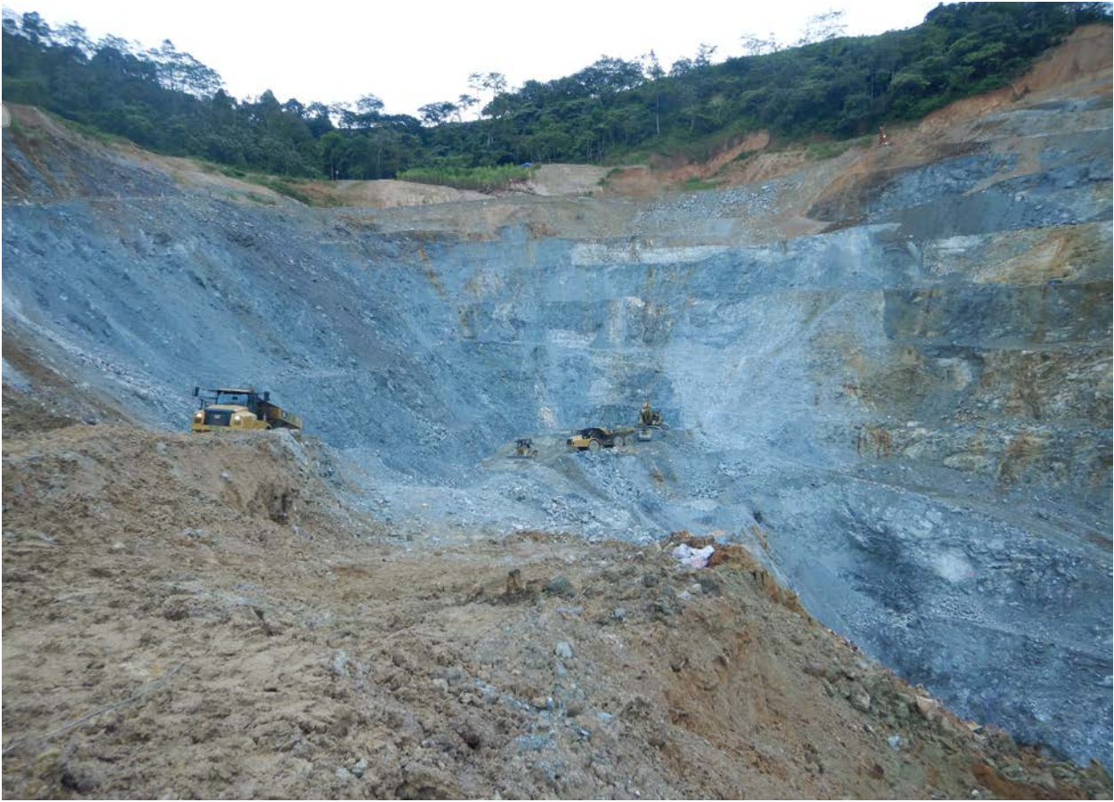
Figure 2: Way Linggo Open Cut Progress looking north at Stage 4 at 31 December 2018
