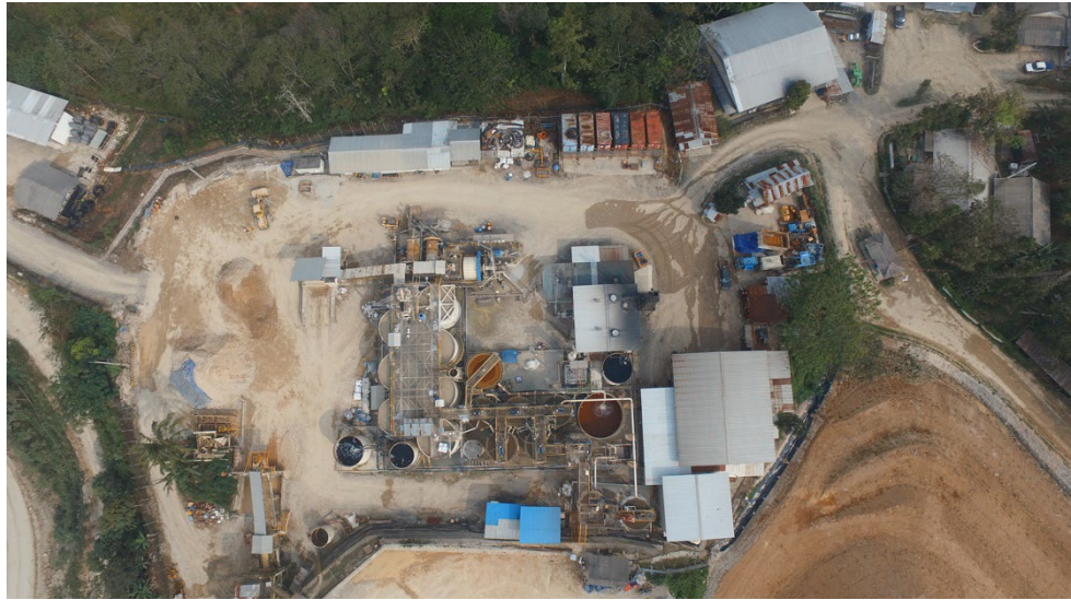
▼ Way Linggo Processing Plant
