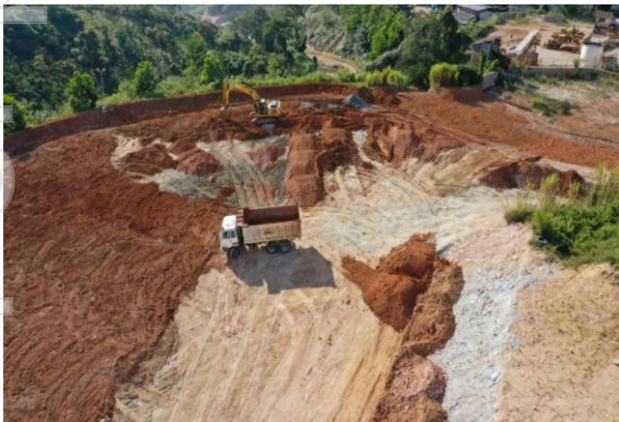
Figures 7 & 8 – Site reclamation activities, reshaping areas, collecting and spreading topsoil and planting
